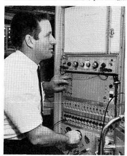
DUANE ARLOWE (7335) demonstrates playback feature of a new Sandia-developed disk recording system. The unit offers a number of advantages in recording shock and impact data over the currently-used tape systems.
